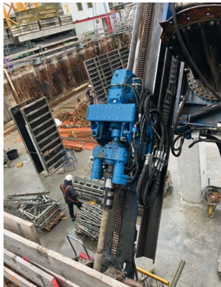
VD150 retraction of hollow bars, 60 m long
